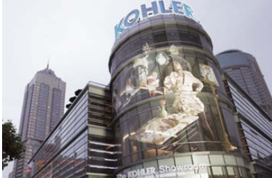
Kohler Design Center opens in Shanghai (China)
